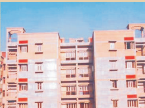
Gurgaon (Phase-I) Housing Scheme : 1088 Flats
