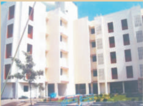
Pune (Ph-II) Housing Scheme : 148 Flats
