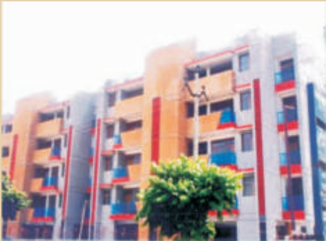
Panchkula (Phase-II) Housing Scheme : 240 Flats
