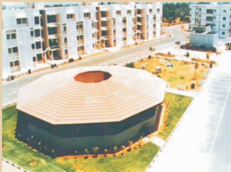
Chennai (Phase-I) Housing Scheme : 524 Flats
