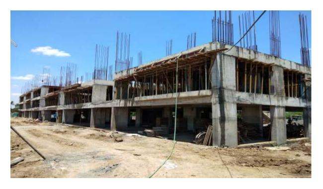
In Block C1Shuttering & Barbending works for Third floor on Progress.
