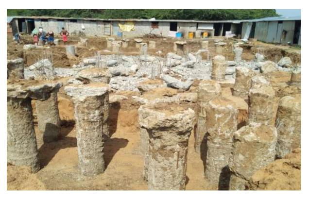
In Block D1 Excavation for Pile cap works, & Barbending for Pile Caps on progress
