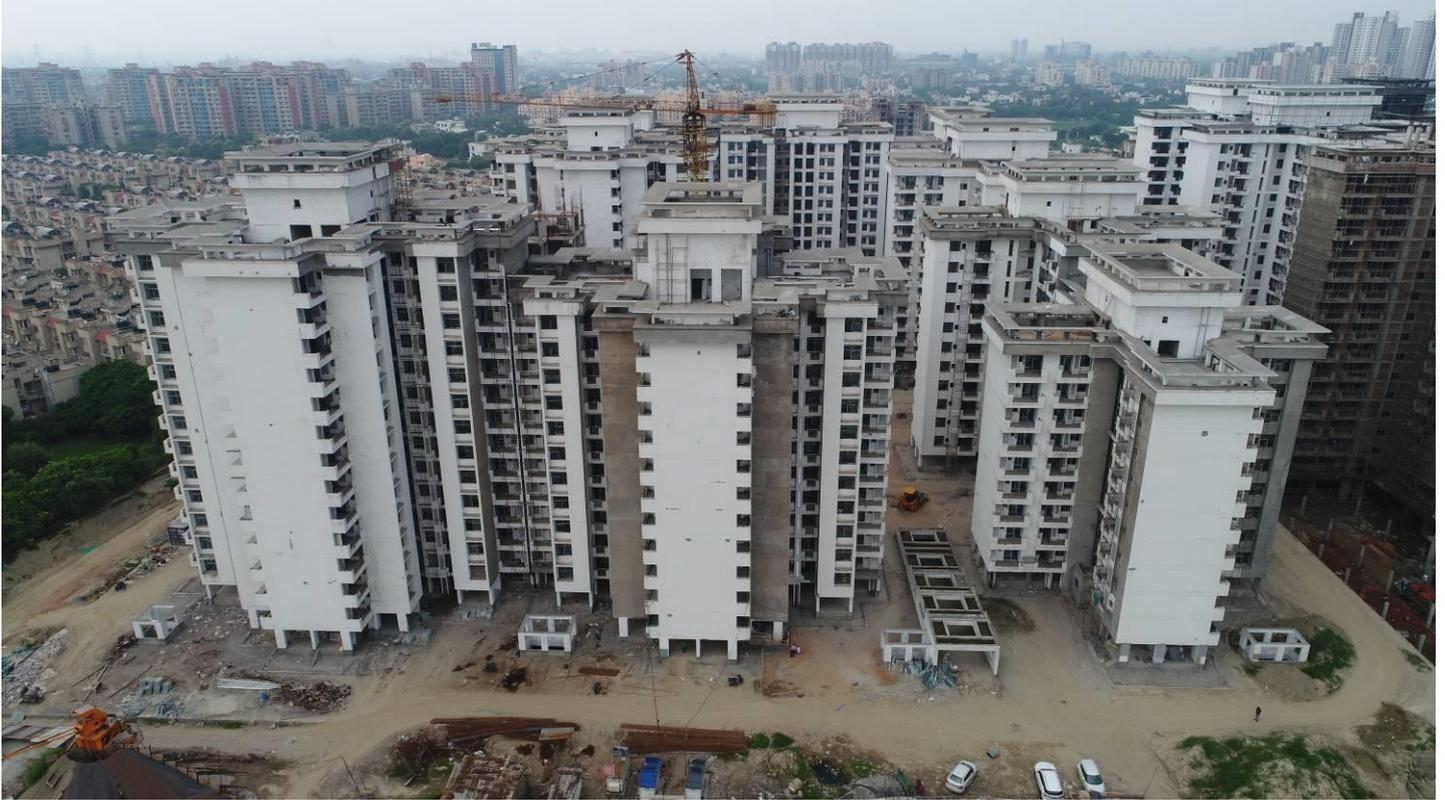
**In Block B-03 11<sup>th</sup> floor Roof slab 75% casted.
