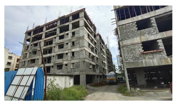
Community Hall: Third Floor level slab concrete casting 100% completed. Column concrete upto Fourth floor level completed. First Floor Finishing works on progress
