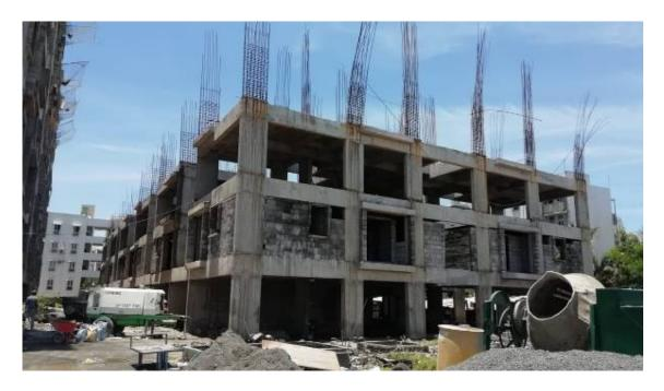
Block C1: Ninth floor level slab First half Concrete casting 100% completed. Slab Shuttering works in 2<sup>nd</sup> Half of Ninth Floor level 25% completed.
