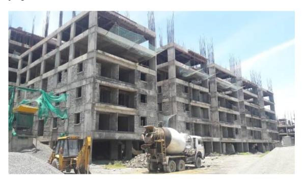
Block D1: Fourth Floor level slab concrete 100% completed. Shuttering & Barbending works for 1<sup>st</sup> half of Fifth Floor level slab 10% completed.
