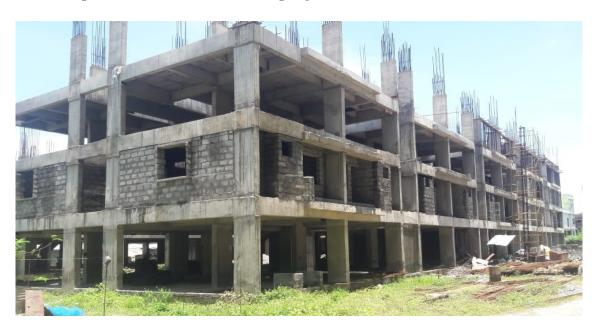
Block A2: Column concrete upto Third floor level 100% completed. Shuttering & Barbending works for 1<sup>st</sup> Half of Third floor level slab 65% completed and balance work on progress.
