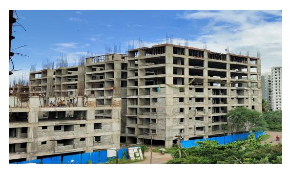
Block D3: Shuttering & Barbending works for 2<sup>nd</sup> Half of Seventh floor level slab 35% completed and balance work on progress.
