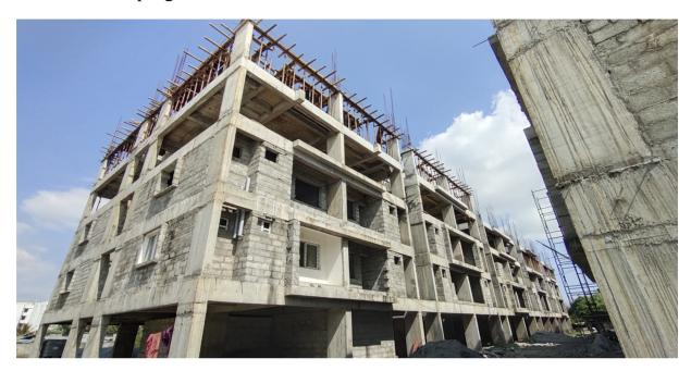
**Block A2:** Fourth floor level slab 1<sup>st</sup> Half Concrete casting 100% completed. Shuttering & barbending works in 2<sup>nd</sup> half of Fourth Floor level slab 50% completed and balance work on progress.
