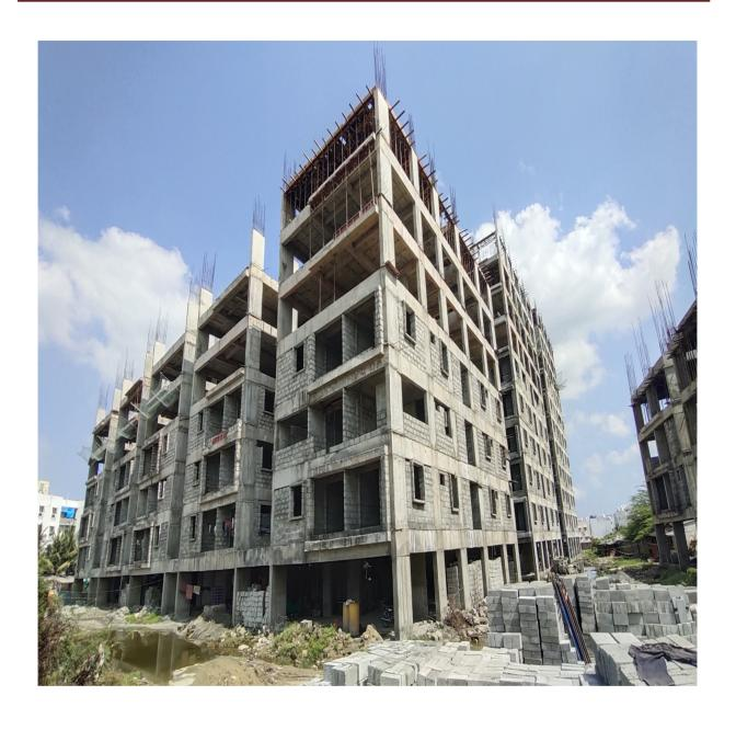
**Block D1:** Sixth Floor level Slab 1<sup>st</sup> half Concrete casting 100% completed. Shuttering & Barbending works for 2<sup>nd</sup> half of Sixth Floor level slab 25% completed and balance works on progress.
