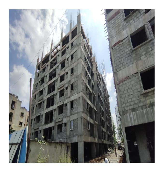
**Community Hall**: Fourth Floor Level slab Concrete casting 100% completed. Columns upto Terrace Floor level 100% completed. Shuttering & Barbending works for Terrace Floor level slab 20% completed and balance works on progress.
