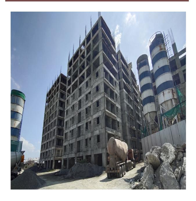
**Block C3:** Shuttering & Barbending works for 1<sup>st</sup> half of Seventh floor level slab 25% completed and balance works on progress.
