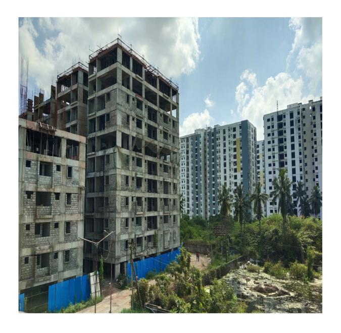
**Block D3:** Columns upto Ninth Floor Level 90% Completed. Shuttering & Barbending works for 1<sup>st</sup> half of Ninth Floor level slab 85% completed and balance works on progress.
