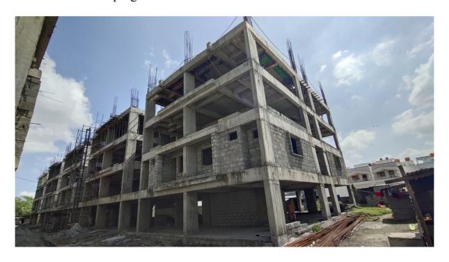
**Block B1:** Terrace Floor Level Slab 1<sup>st</sup> half concrete casting 100% completed. Shuttering and Barbending works for 2<sup>nd</sup> half of Terrace floor level slab 50% completed and balance work on progress.
