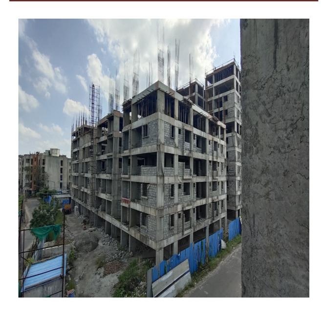
Block D2: Columns upto Terrace floor level 85% completed. Shuttering & Barbending works for 1st half of Terrace Floor level slab 60% completed and balance works on progress.
