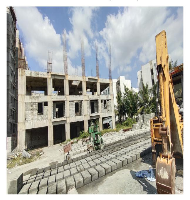
**Block C1:** Columns upto Terrace Floor level 50% completed. Shuttering & Barbending works in 1<sup>st</sup> half of Terrace Floor level slab 20% completed and balance works on progress.
