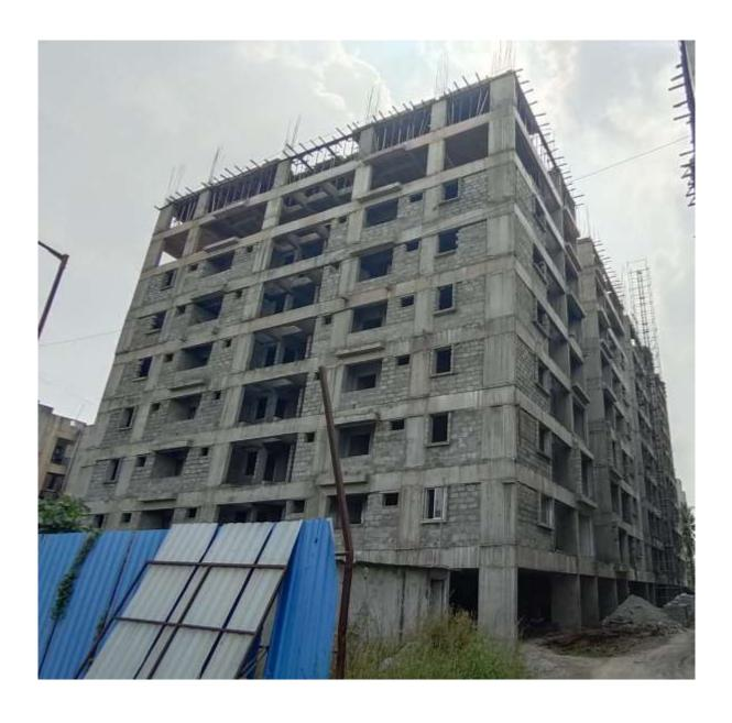
**Community Hall**: Columns upto Terrace Floor level 100% completed. Shuttering & Barbending works for Terrace Floor level slab 50% completed and balance works on progress.
