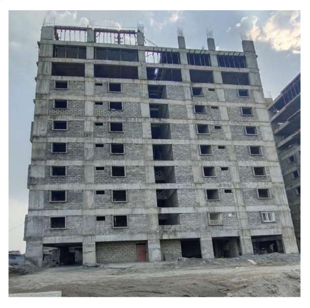
**Block C2:** Shuttering & Barbending works for 2<sup>nd</sup> half of Tenth floor level slab 50% completed and balance works on progress.
