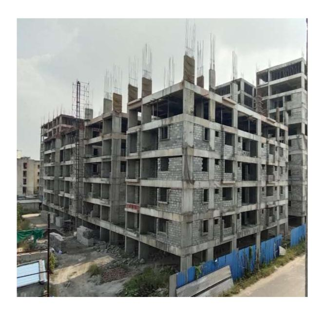
**Block D2:** Terrace Floor level Slab 1<sup>st</sup> half Concrete casting 100% completed.
