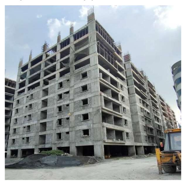
**Block C3:** Shuttering & Barbending works for 1<sup>st</sup> half of Seventh floor level slab 50% completed and balance works on progress.
