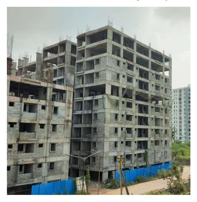
**Block D3:** Ninth Floor level Slab 1<sup>st</sup> half Concrete casting 100% completed. Shuttering & Barbending works for 2<sup>nd</sup> half of Ninth Floor level slab 45% completed and balance works on progress.
