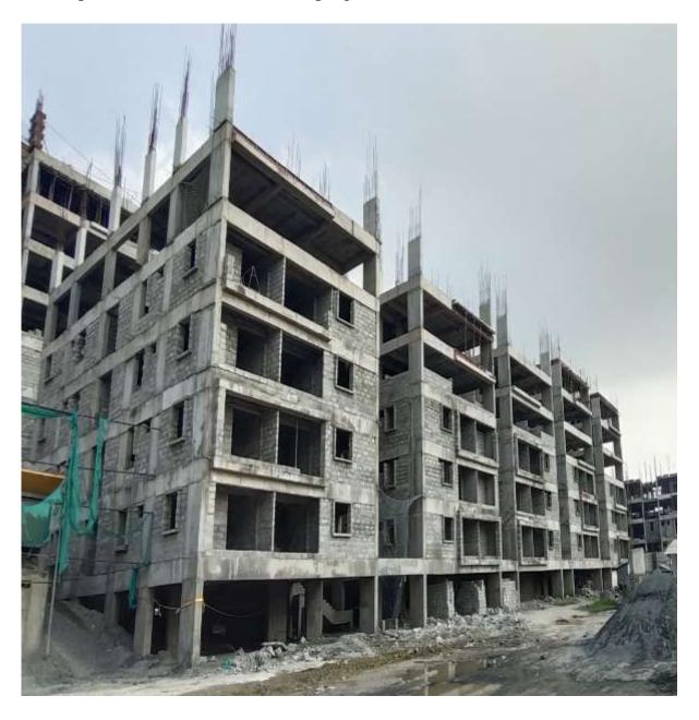
**Block D1:** Sixth Floor level Slab 1<sup>st</sup> half Concrete casting 100% completed. Shuttering & Barbending works for 2<sup>nd</sup> half of Sixth Floor level slab 85% completed and balance works on progress.
