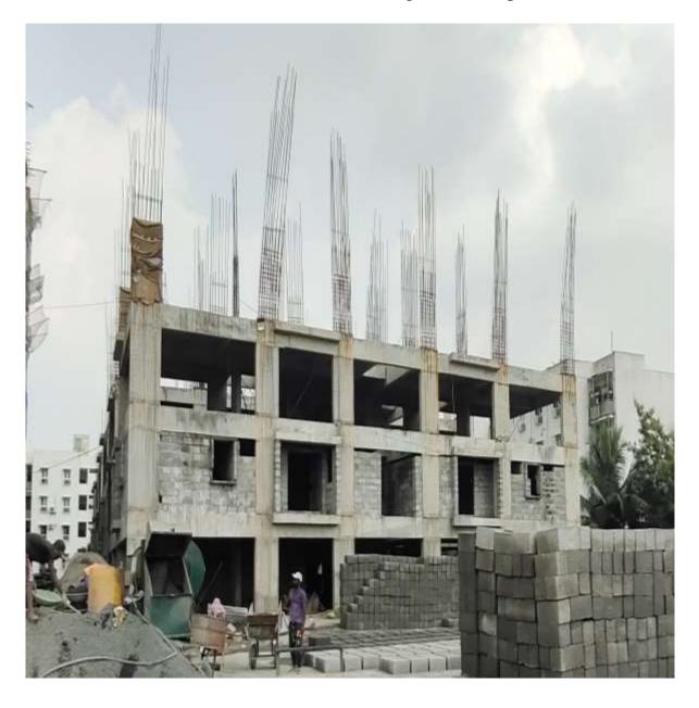
**Block C1:** Columns upto Terrace Floor level 100% completed. Shuttering & Barbending works in Terrace Floor level slab 50% completed and balance works on progress.
