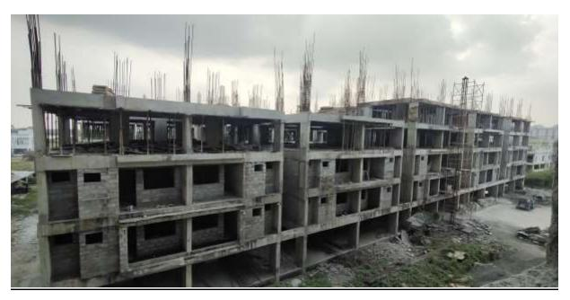
**Block A2:** Shuttering & barbending works in 2<sup>nd</sup> half of Fourth Floor level slab 60% completed and balance work on progress.
