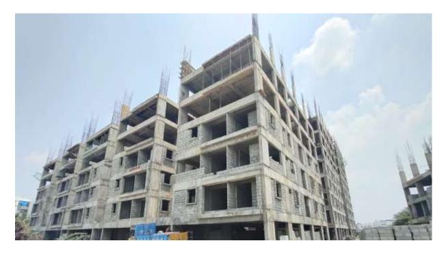
Block D1: Fifth Floor level slab First half concrete 100% completed. Shuttering & Barbending works for 2<sup>nd</sup> half of Fifth Floor level slab 15% completed.
