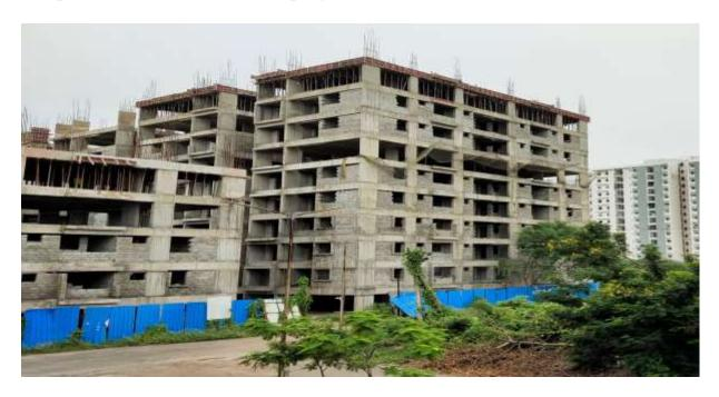
Block D3: Seventh Floor Level slab concrete casting 100% completed. Shuttering & Barbending works for 1<sup>st</sup> Half of Eight floor level slab 50% completed and balance work on progress.
