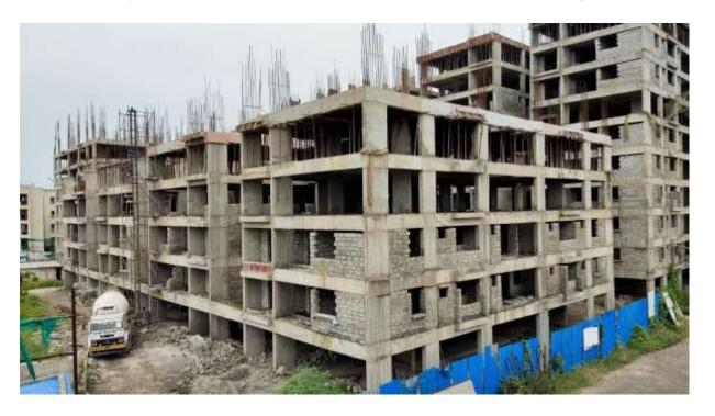
Block D2: Tenth Floor Level slab First Half concrete casting 100% completed. Shuttering & Barbending works for 2<sup>nd</sup> Half of Tenth floor level slab 10% completed and balance work on progress.
