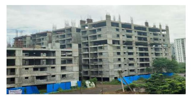
Block D3: Eight Floor Level slab 1<sup>st</sup> half concrete casting 100% completed. Shuttering & Barbending works for 2<sup>nd</sup> half of Eight floor level slab 25% completed and balance work on progress.
