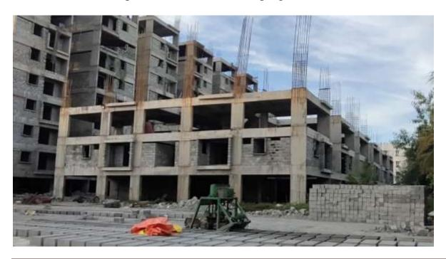
Block C1: Ninth floor level slab Concrete casting 100% completed. Shuttering & Barbending works in 1<sup>st</sup> Half of Tenth Floor level 95% completed.
