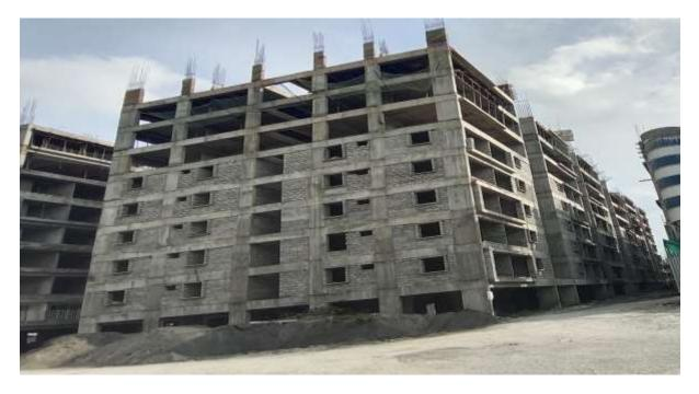
Block C3: Sixth Floor level slab concrete 100% completed. Column upto Seventh floor level 80% completed.
