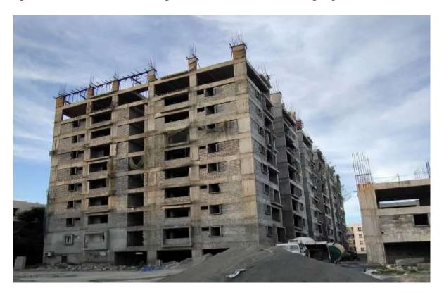
Block B2: Third Floor Level slab concrete casting 100% completed. Bar bending works for Columns up to fourth floor level on progress.
