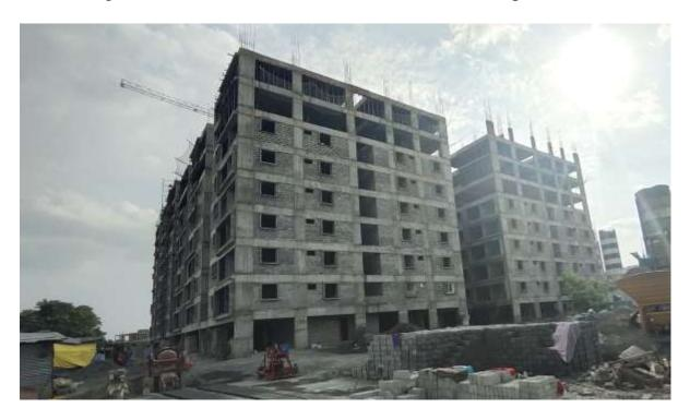
Block C2: Shuttering & Barbending works for 2<sup>nd</sup> Half of Ninth floor level slab 50% completed and balance work on progress. Columns upto Tenth Floor level 50% completed.
