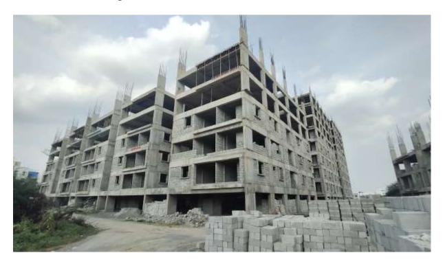
Block D1: Shuttering & Barbending works for 2<sup>nd</sup> half of Fifth Floor level slab 100% completed. Columns upto Sixth floor level 45% completed.
