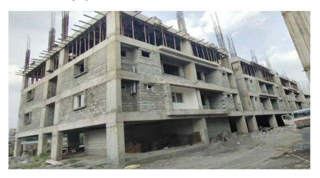
Block A2: Third floor level slab 1<sup>st</sup> half concrete 100% completed. Shuttering & barbending works in 2<sup>nd</sup> half of Third Floor level slab 70% completed and balance work on progress.
