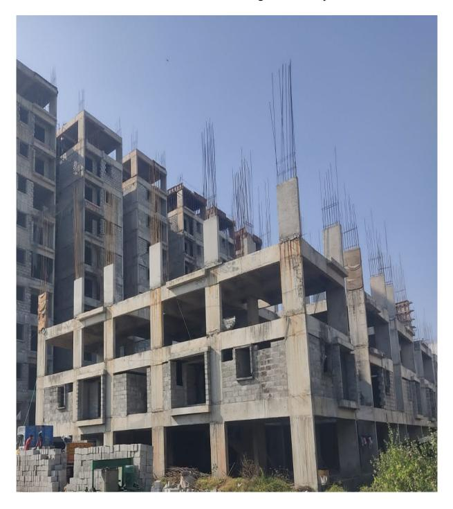
**Block C1:** Columns upto Terrace Floor level 100% completed. Shuttering works in Terrace Floor level slab 100% completed and Barbending works on progress.
