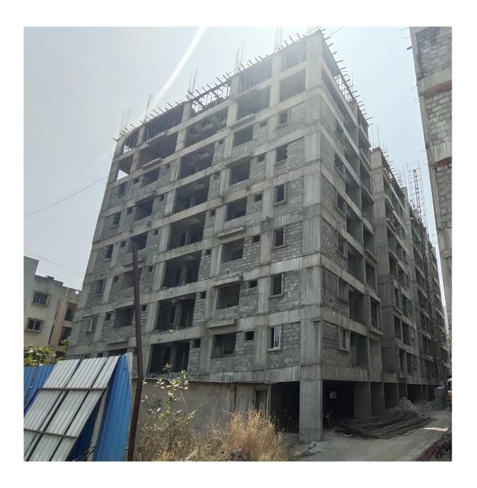
**Community Hall**: Columns upto Terrace Floor level 100% completed. Shuttering & Barbending works for Terrace Floor level slab 95% completed and balance works on progress.
