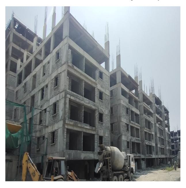
**Block D1:** Sixth Floor level Slab Concrete casting 100% completed. Shuttering & Barbending works for 1<sup>st</sup> half of Seventh Floor level slab 75% completed and balance works on progress.
