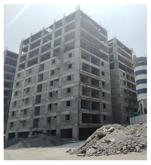
**Block C3:** Seventh floor level slab First half Concrete casting 100% completed.
