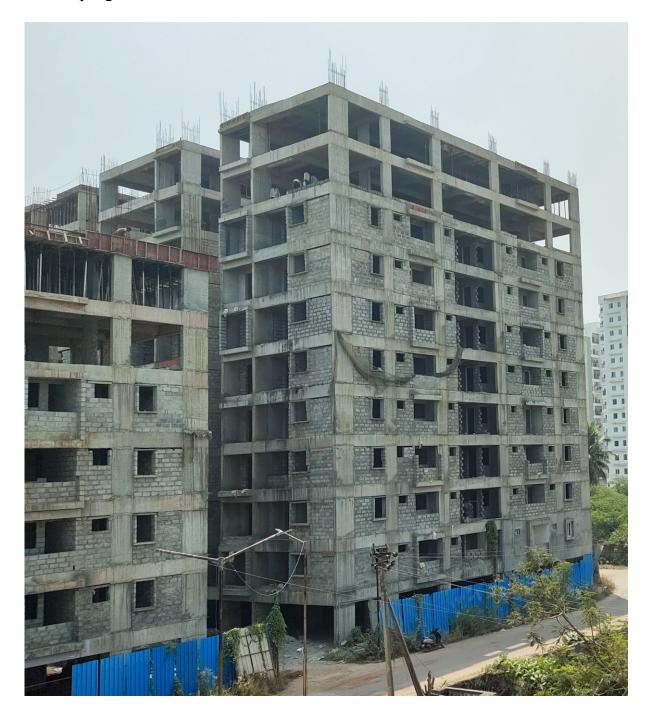
**Block D3:** Ninth Floor level Slab 1<sup>st</sup> half Concrete casting 100% completed. Shuttering & Barbending works for 2<sup>nd</sup> half of Ninth Floor level slab 45% completed and balance works on progress.
