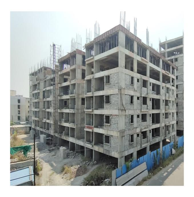
**Block D2:** Terrace Floor level Slab 1<sup>st</sup> half Concrete casting 100% completed. Shuttering works for 2<sup>nd</sup> half of Terrace floor slab 75% completed and balance works on progress.
