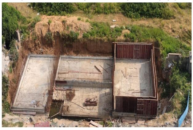
**Sewage Treatment Plant- 1**: Base slab RCC 100% completed.
