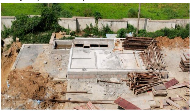
U.G Sump- 2: Base slab RCC 95% completed. Wall shuttering and bar binding in progress
