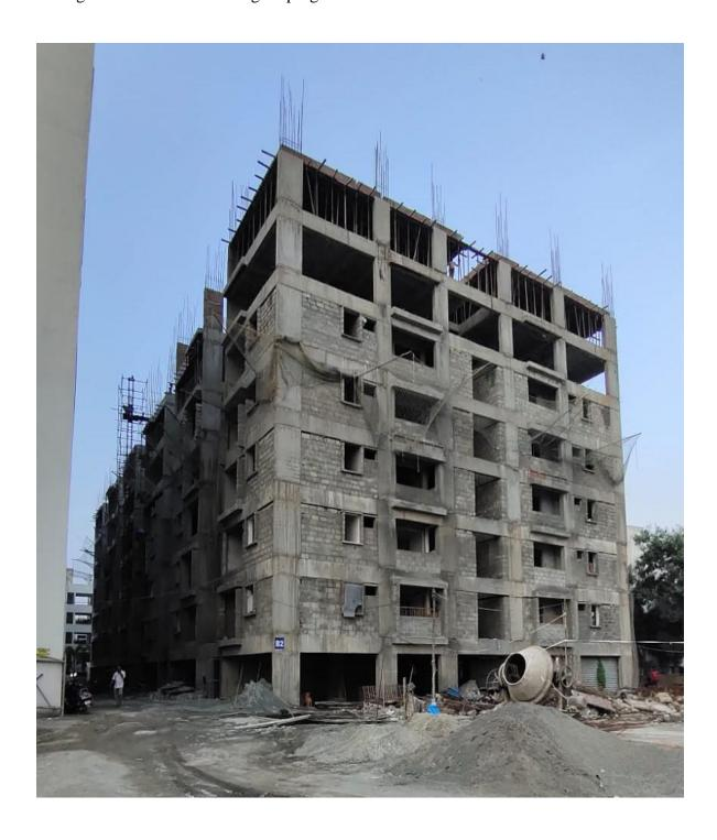
**Block C1:** External Plastering overall 95% completed. 2<sup>nd</sup> Coat of Primer 95% completed. Lift Installation works on Progress. Terrace weathering course work 90% completed.
