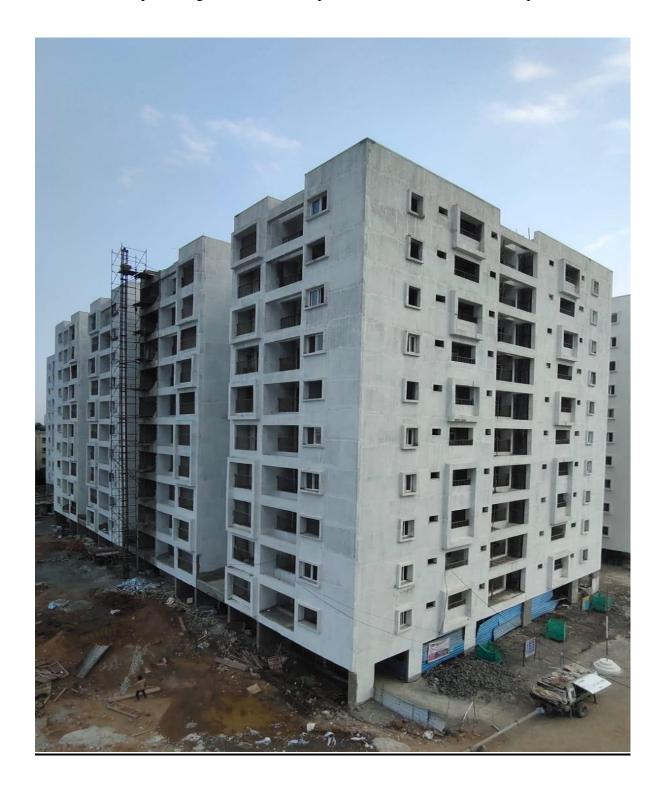
**Block D2:** Over Head Water Tank 100% completed. Lift installation works on progress. Terrace weathering course on progress. External Painting works on progress.
