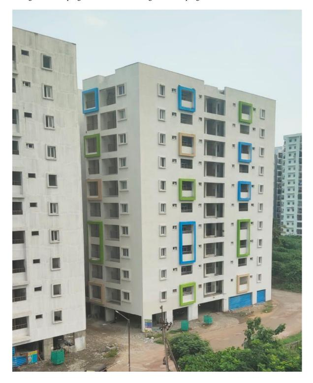
**Block D3:** External Plastering work overall 95% completed. 1<sup>st</sup> Coat of Primer 95% completed. Tiling works on progress.
