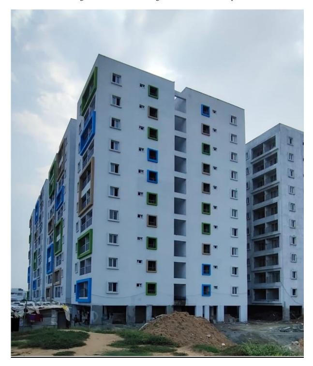
**Block C2:** External plastering overall 95% completed. 1<sup>st</sup> Coat Primer 95% completed. Lift Erection works on Progress. Terrace weathering course work 50% completed.
