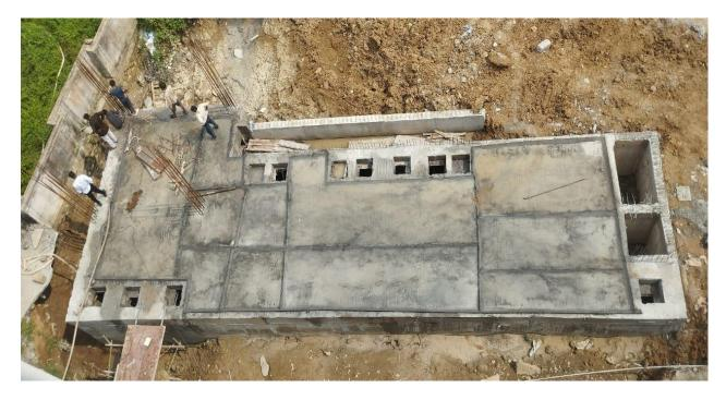
U.G Sump 1 (Near D Block) – Base Slab RCC 95% completed. Sump wall & Top Slab Concrete 100% completed.
