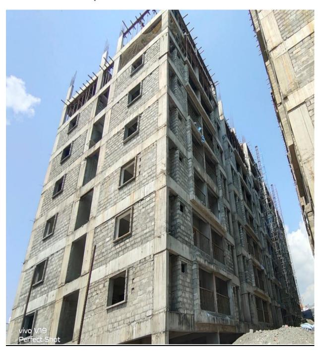
**Block B1:** External Plastering South side elevation 100%, East side 80%, West Side 90% & North Side 90% completed.
