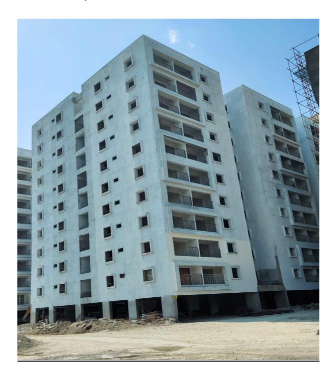
**Block C3: Terrace Floor level slab** Concrete casting 100% completed. Terrace floor columns concrete 100% completed.
