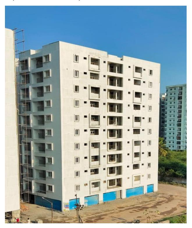
**Block D3: Terrace** Floor level slab Concrete casting 100% completed. External Plastering work overall 95% completed. 1<sup>st</sup> Coat of Primer 75% completed.
