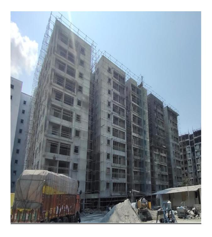
**Block D1: Terrace** Floor level slab Concrete casting 100% completed. External plastering in West side 90% completed, North side 20% completed, South side 30% completed and balance works on progress.
