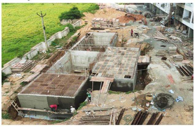
U.G Sump- 2: P.C.C for Base Slab completed. Barbending works for Base slab on Progress.
