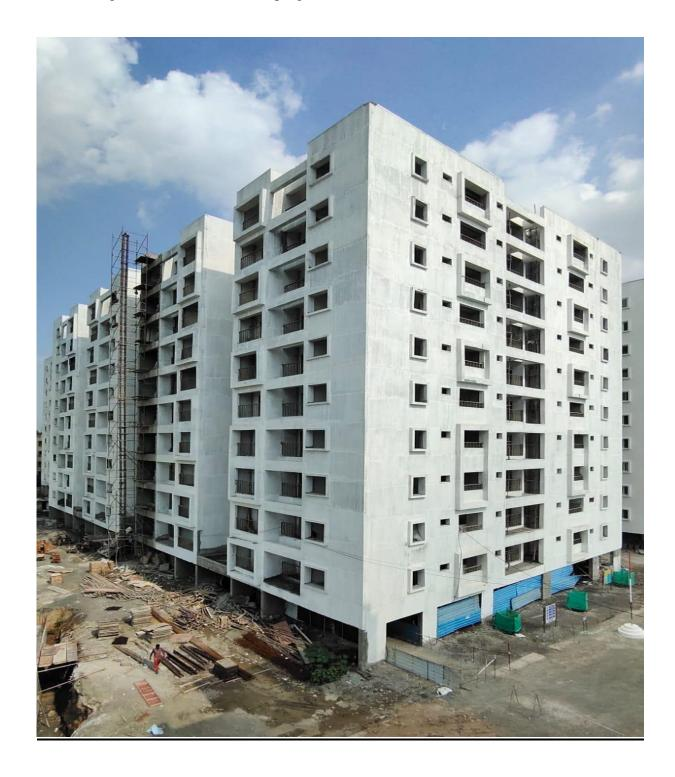
**Block D2:** Lift installation works 80% completed. Terrace weathering course 85% completed. O.H.T Water proofing works on progress.
