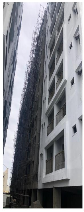
**Block B1:** Lift Installation works 90% completed Fixing of UPVC Windows 90% completed. Terrace Weathering course 95% completed.
