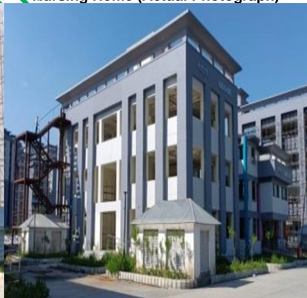
Nursing Home (Actual Photograph)
