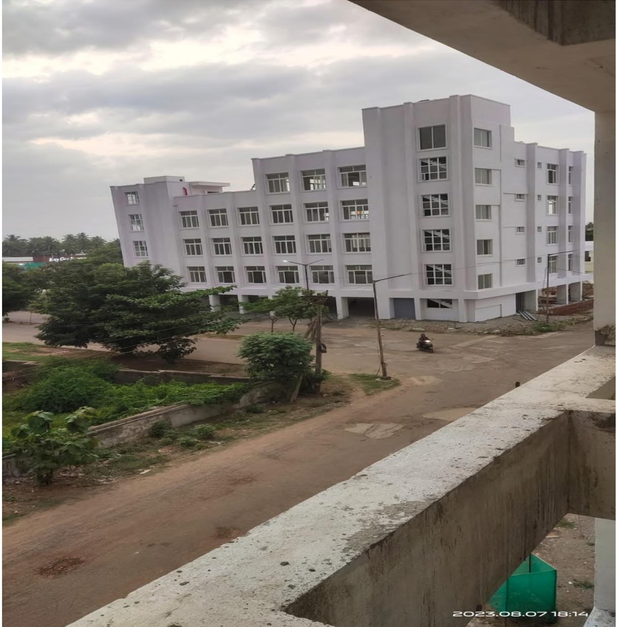
**Block A1:** Parapet columns 100% completed .External plastering in West side 95% completed, North side 40% completed & East side 45% completed.
