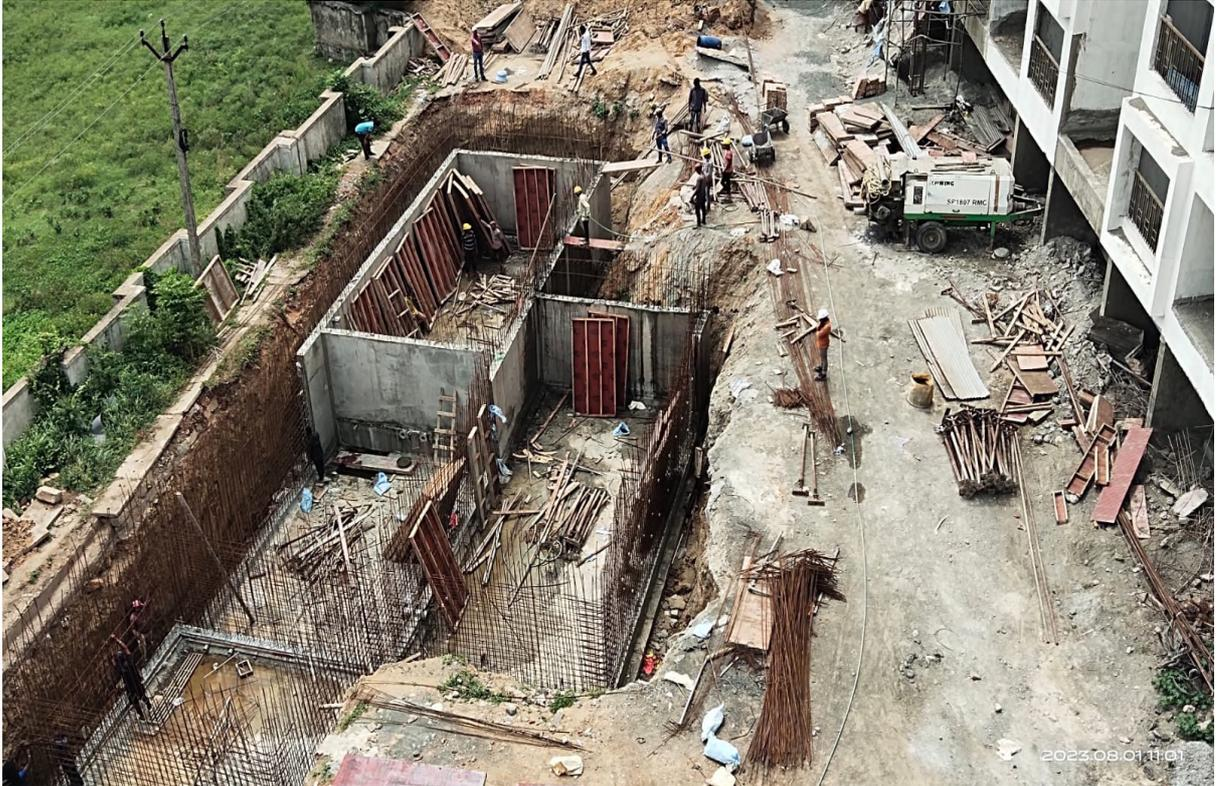
**Underground Sump at B1-Block – P.C.C 100% completed.**
