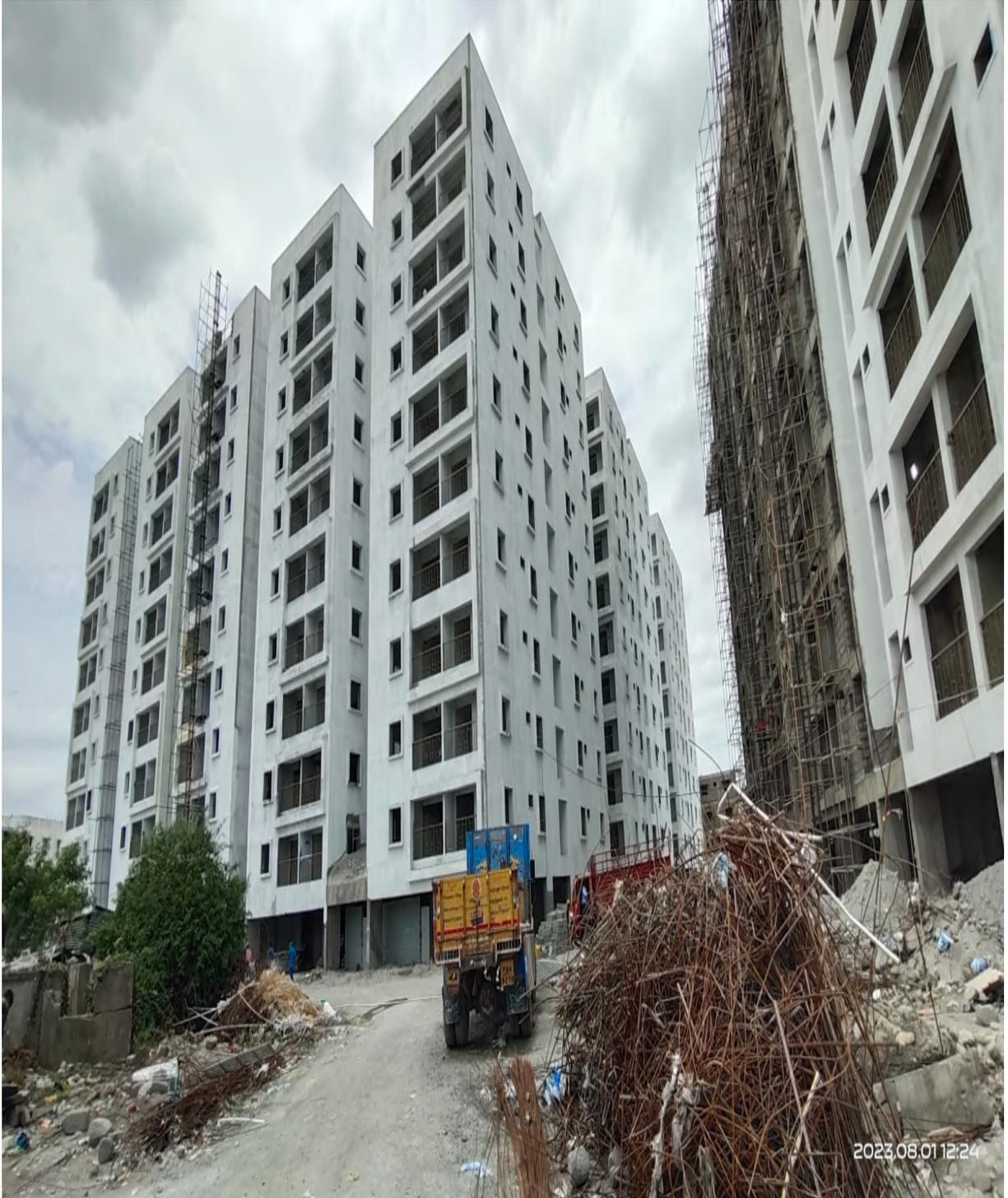
**Block D1:** External plastering overall 95% completed. 1<sup>st</sup> Coat Primer 95% completed. Internal Plumbing lines 90% & Sanitary Lines 35% completed .
