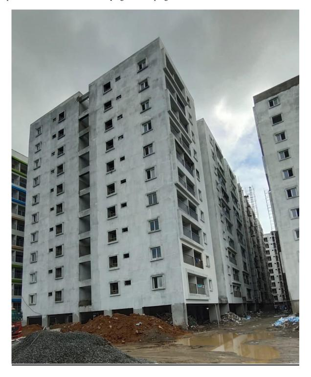
**Block C3:** External Plastering completed. Fixing of UPVC Windows & Laying of Floor Tiles on progress.
