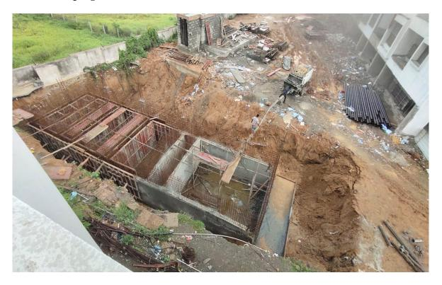
Sump 1 – Base Slab RCC 95% completed. Sump wall Concrete 40% completed and balance works on progress.
