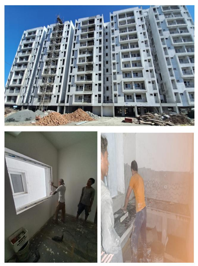
**Block A1:** Fixing of UPVC Windows, laying of Kitchen Granite counter on progress.
