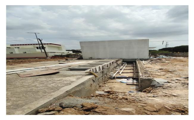
Sewage Treatment Plant 1 (Near C Block). Base slab RCC completed. Reinforcement works for Wall 85% completed.
