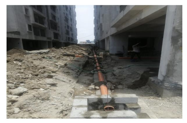
Excavation works around C3 block on progress. Connection of Sewer line to Chamber & plastering on progress.
