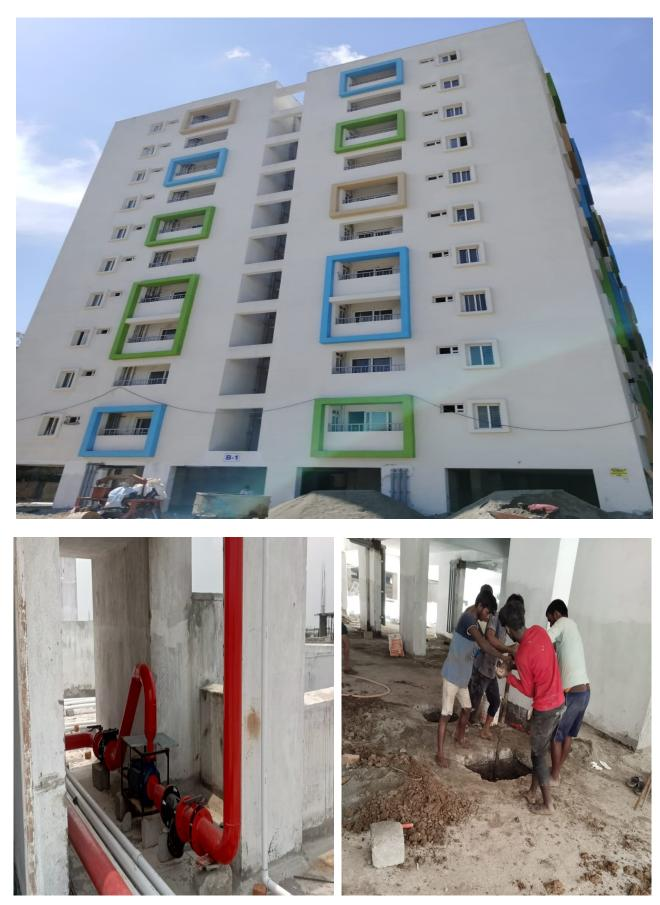
Block B1: Firefighting Pump installation completed. Earth pit for Lifts on progress.
