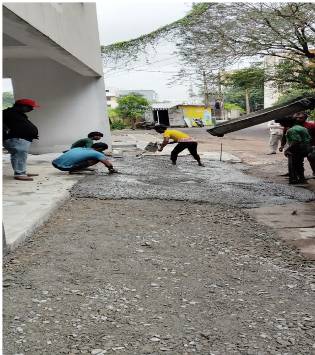
Block D3: Laying of PCC around the block on progress.
