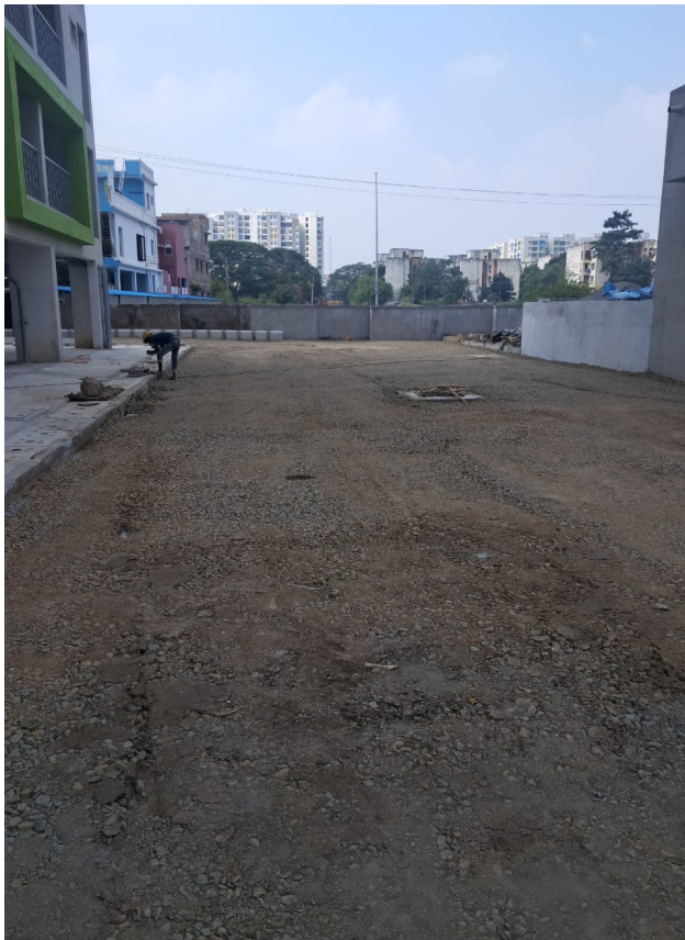
Road Works : Laying of Granular Sub base in A1 North side completed.
