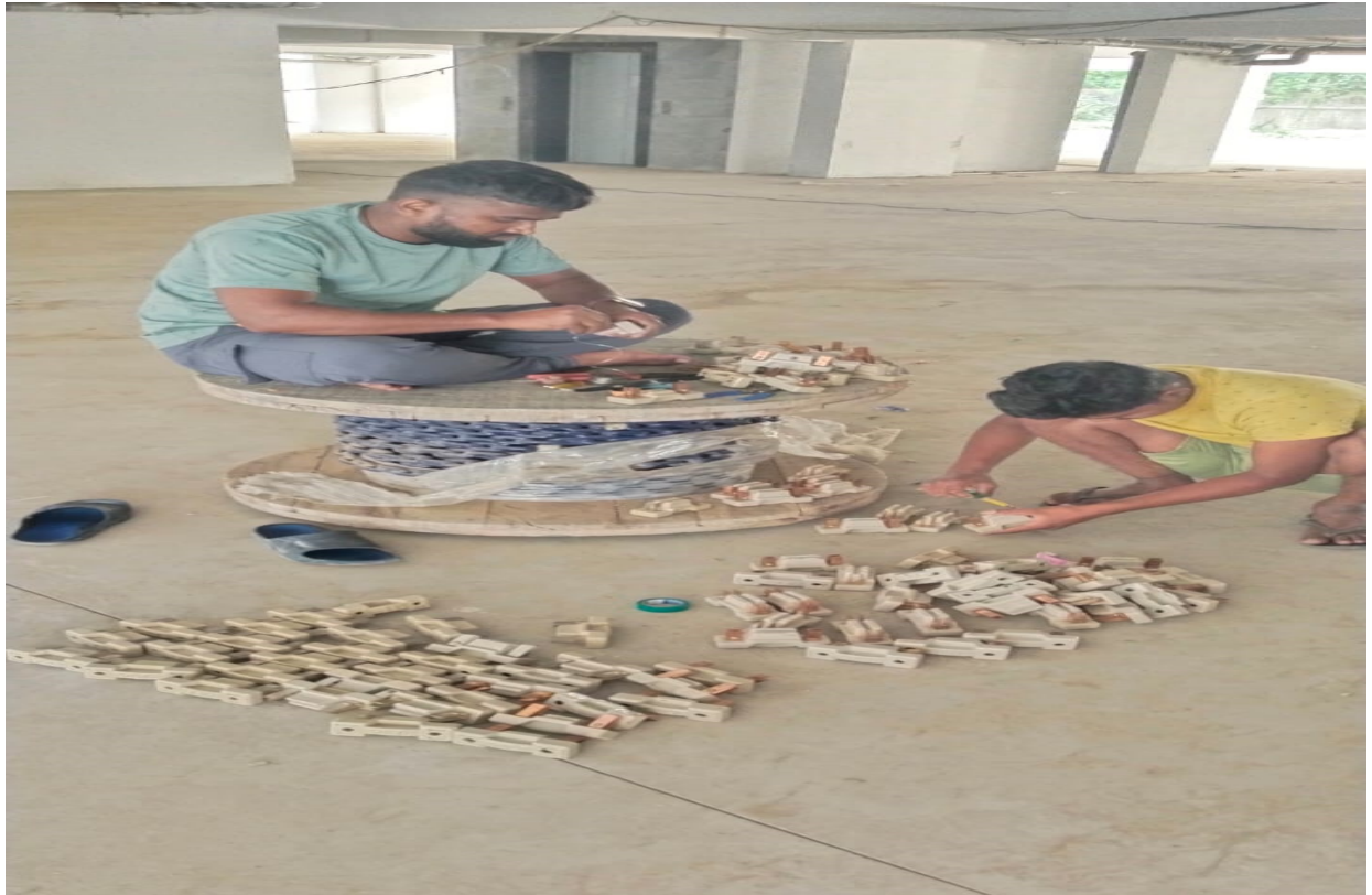
Block D2: Fixing of fuses in E.B Panel on progress
