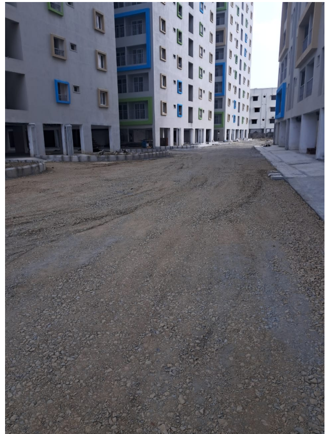
Road Works : Laying of Granular Sub base in A1 North side completed.
